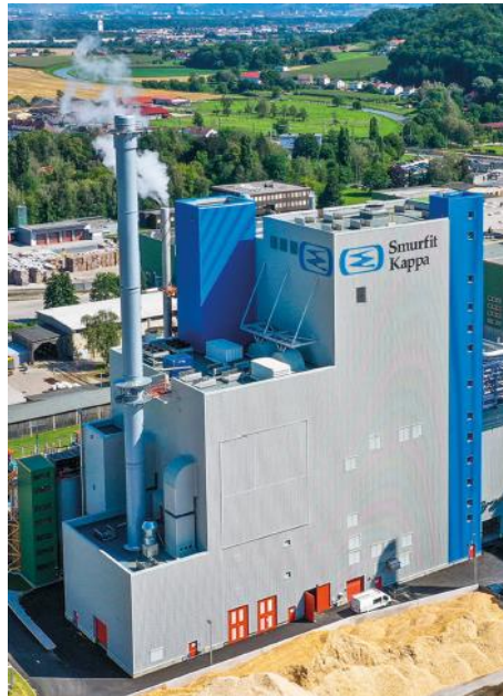
SKN Nettingsdorf Black Liquor Boiler (2020)
